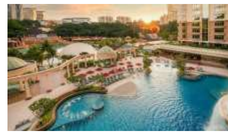
Sunway Resort Hotel Refurbishment
