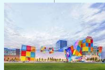
Sunway Carnival Mall Existing Wing
